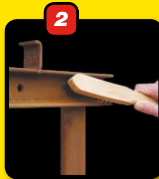
2 Manually derusting and degreasing
