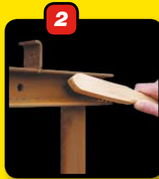
2 Manually derusting and degreasing
