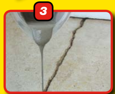
3 Pour mixture in the crack and level off with scraper
